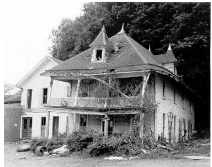
Newport House in 1984 - lb photo
